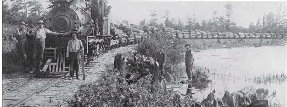
Shay's locomotive allowed logging companies to transport felled timber more effectively. Pictured here is a Shay used by the lumber company Murphy & Diggins in Cadillac, Michigan. (Photo courtesy of the Claude Thomas Stoner Photographs and Papers, Bentley Historical Library, HS15724.)
